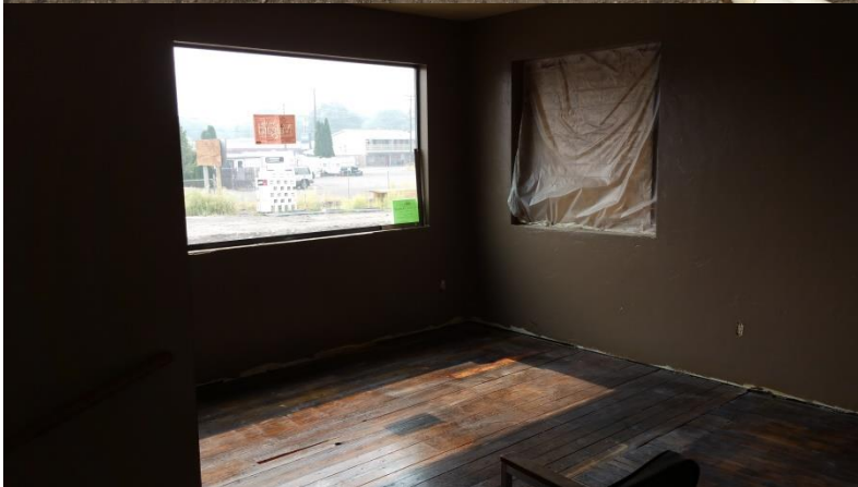
Construction of Hines Meat Company
